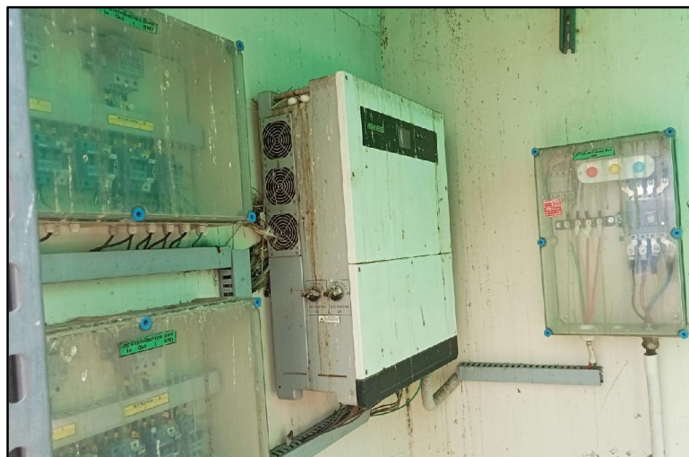
Solar Panels on rooftop
